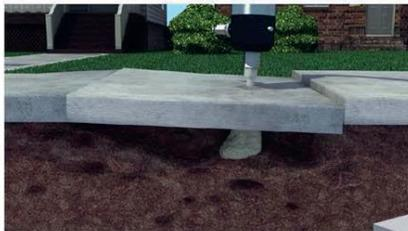
Two parts of the polyurethane foam travel down a set of hoses separately and mix in the nozzle. They pass through the port and slab in liquid form.
